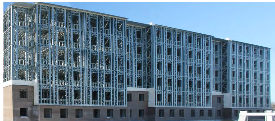
Multi-storey (up to 6) residential and social buildings with cold roll-formed galvanized steel framing (STEELTOWN® series)
