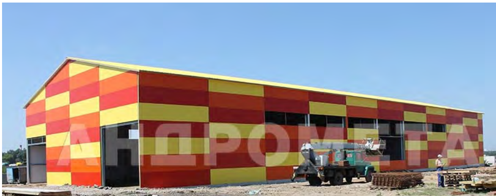
Commercial buildings with cold roll-formed galvanized steel frames (STERK® series)
